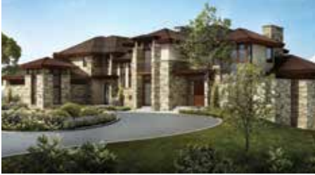
Breathtaking 6,300 s.f. concept home Valley's Edge received top honors—A Crystal Key Award for Innovation and Design and the Gold Key Award for Excellence in New Construction.
