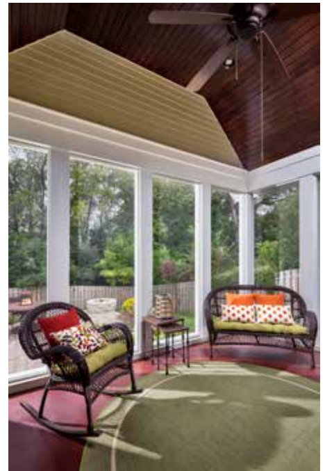
1x4 v-groove pine on ceiling in mahogany finish. Floors are stained concrete.
