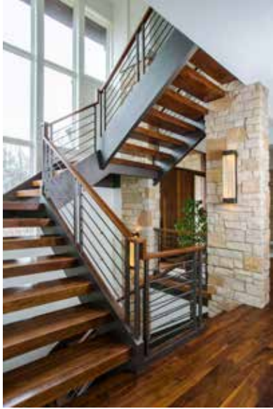
Floating, open tread, 3"x12" walnut staircase with interior stone columns.
