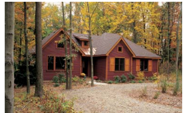
One of the many cottages completed at Stone's Throw
