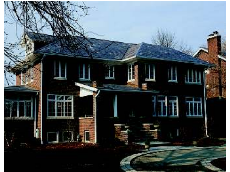
▲ New tuckpointing, a restored slate roof, and a new driveway highlight the front exterior of the Turn of the Century House.
