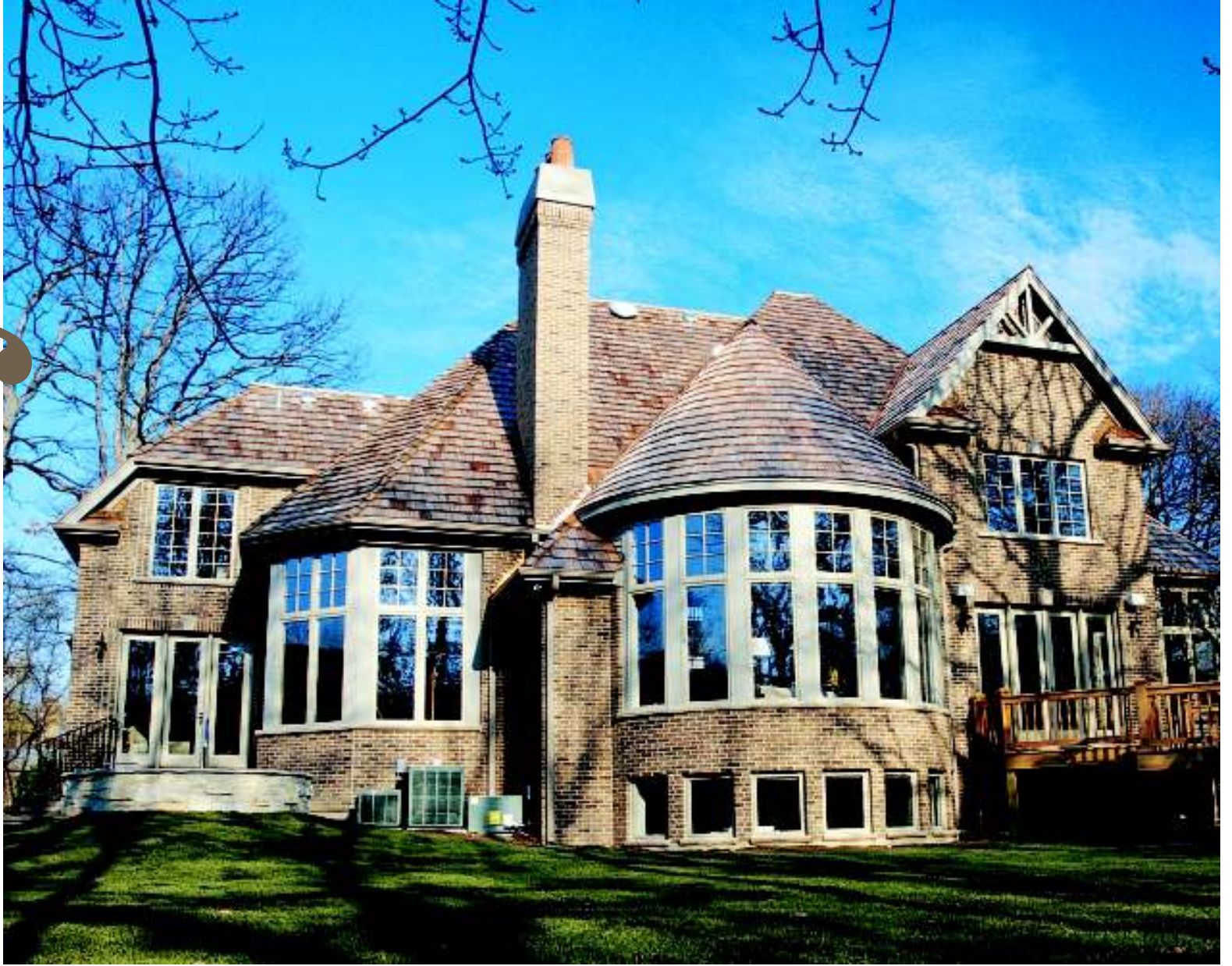
▲ The rear view of The Transition House, with its spa to the left, deck to the right, and plenty of windows in between!
