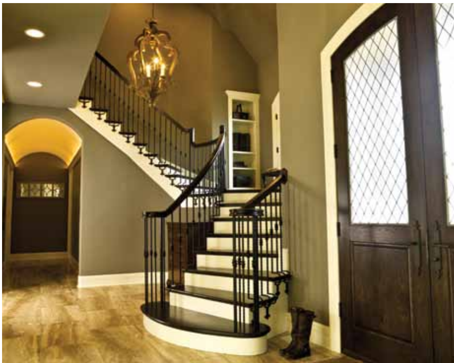
The open staircase with its custom metal balustrade wrapping the stair treads.
